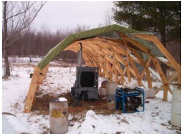
**VeggieGen, Part 2 -- The completion of the project. VG is shown above in the framed but uncovered GeoQuon at the Spence homestead.**
